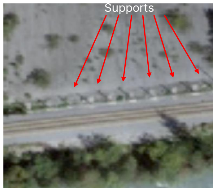
Figure 5-50: Rockfall net support posts
